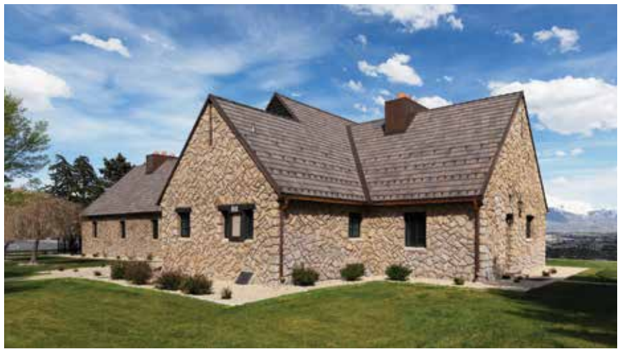
Camp Williams Officers Club after renovation, May 24, 2023.
