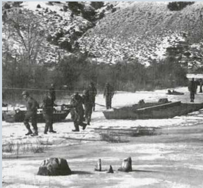
Members of the 1457th Engineer Battalion, 19th Special Forces Group (Airborne), 163rd Armored Cavalry Regiment, and 140th Field Artillery assisted in channel clearing, water supply protection, roadway repair and dike construction in Utah County.
