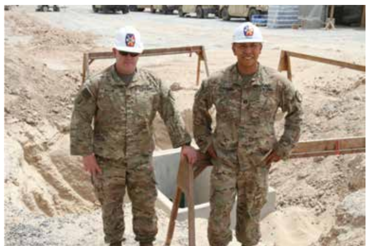
Maj. Corey Mellor (left), projects manager for the 65th Field Artillery Brigade, and Capt. James Redhouse (right), deputy project manager for the 65th Field Artillery Brigade, pose for a photograph in front of a manhole Aug. 8, 2018, at Camp Redleg, United Arab Emirates. The manhole is part of an ongoing project to upgrade the camps internet connectivity.
