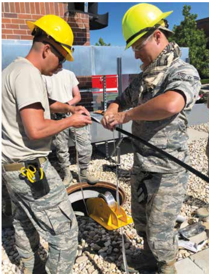
Tech. Sgt. Martin Montano (left) and Airman 1st Class Shane Miller pull fiber-optic cable to support communications and alarms for the munitions storage area at Gowen Field, Idaho.
