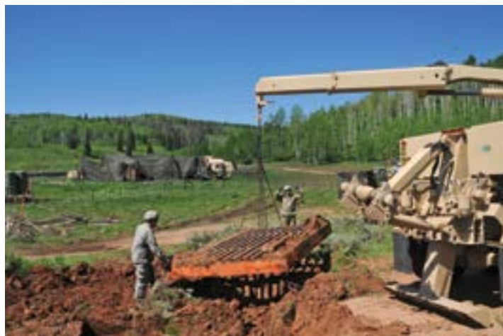
Soldiers with the Forward Support Company, 1457th Engineer Battalion remove a cattle guard as part of upgrades to Mud Creek Road at Strawberry Reservoir, June 8. The roadwork is part of an interagency project between the Utah National Guard and the U.S. Forest Service allowing Utah Soldiers to train realistic, disaster-response operations while improving community recreation facilities. Soldiers with the 116th Engineer Company, 1457 Engineer Battalion excavate and prep the ground as part of upgrades to Mud Creek Road at Strawberry Reservoir, June 8.
