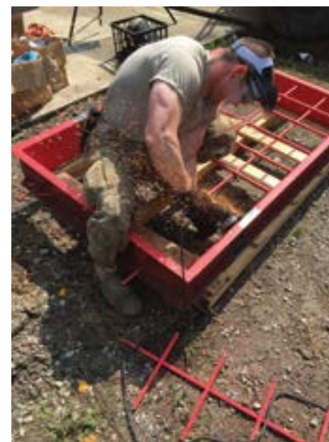
Staff Sgt. J.D. Williamson, 19th Group Support Battalion, grinds a window after making modifications.
