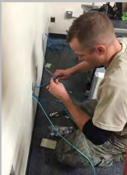
Left to right: Tech. Sgt. Austin Walje terminating CAT6 wire at Boise Idaho Air National Guard Base. Staff Sgt. Charles Treutlein and Senior Master Sgt. Michael Perez certifying on tower climbing during a preventative-maintenance inspection at Portland Air National Guard Base. Relocation team with 130th EIS at Joint Space Operation Center Launch and Test Range, Vandenberg Air Force Base.
