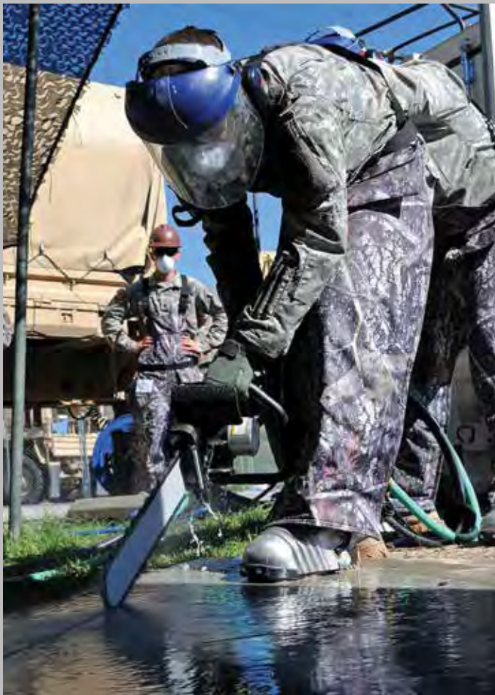
Spc. Kevin Gwilliam from the 624th Engineer Company, 1457 Engineer Battalion, uses a wet saw to cut a section of concrete as part of a renovation project on a restroom facility at the Renegade Point Marina, Strawberry Reservoir, June 8.
