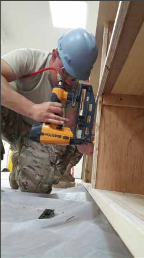
Structures Apprentice, Senior Airman Cody Schmidt, works on the finishing carpentry of a hand-built counter for a post office at an undisclosed location in Southwest Asia.
