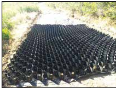
Geoweb placement on the north boundary trail.
