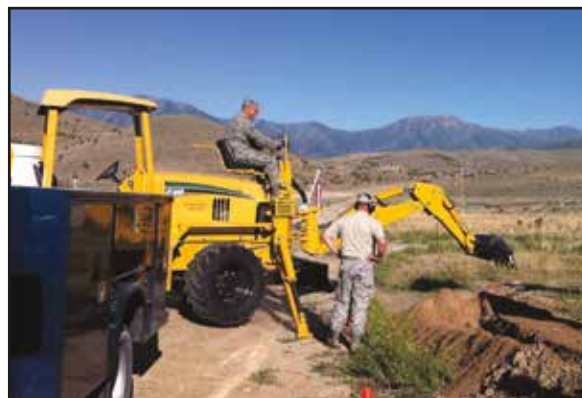
Senior Airman Adam Farley completes a fiber installation project while deployed to the Persian Gulf. Members of the 130th work on a project to bury conduit for seven miles of fiber-optic cable to connect Camp Williams ranges.
