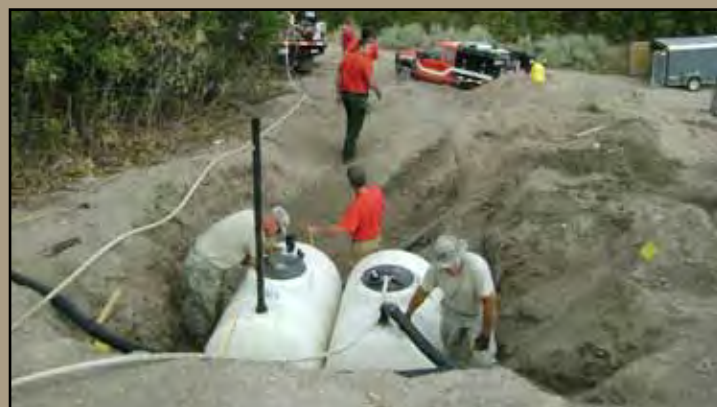
Water tanks are placed for "wildlife guzzler."
