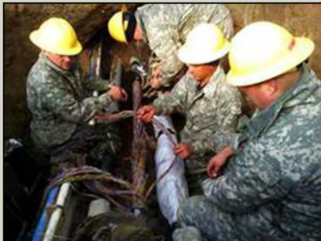
Left to right: A team from the 130th installs an antenna as part of a practice Operational Readiness Inspection. Members of the 130th Engineering Installation Squadron repair three major cables containing over 8,000 phone lines at Mountain Home Air Force Base, Idaho. Unit members complete a cable splice during the 130th's Operational Readiness Inspection exercise.
