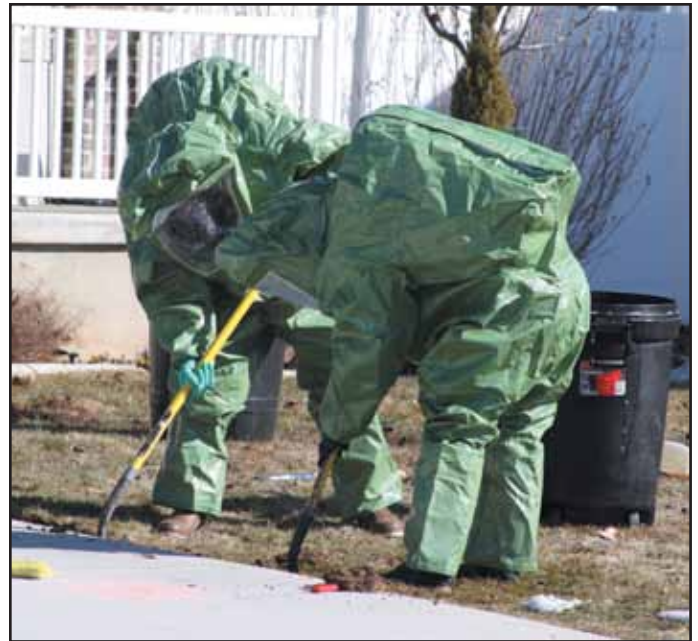
Layton firefighters dig up phosphine gas-emitting pellets placed under the driveway by an exterminator.
